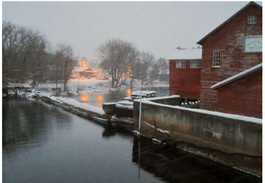
The Croghan Island Mill is more than 100 years old. It's one of the last commercially operating water-powered sawmills. Wedged between two crumbling dams on the Beaver River, the mill will be forced to close if those dams are not replaced. The Department of Environmental Conservation already removed some of the most damaged stop logs last summer.
